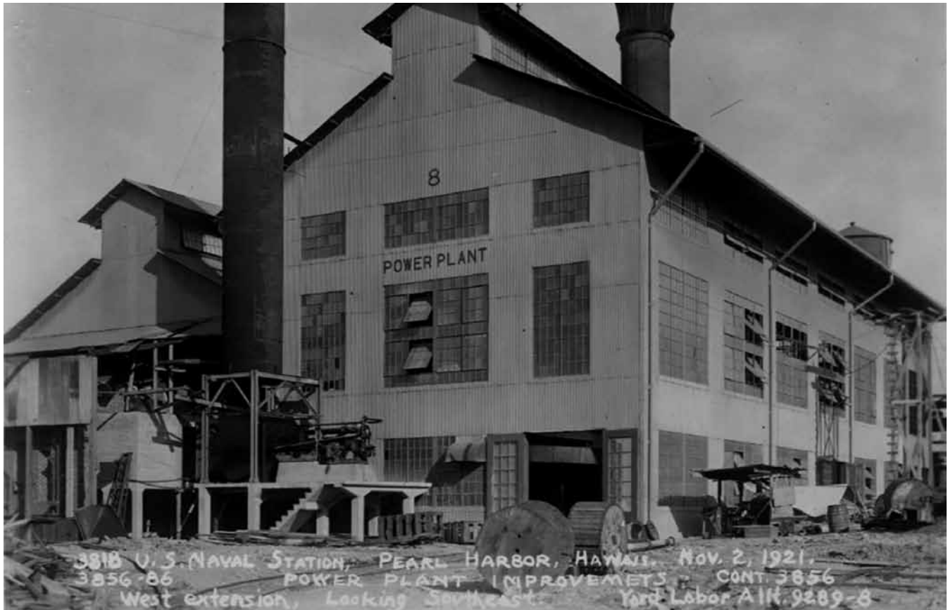
Building 8 is the historic power plant for the Pearl Harbor Naval Shipyard.
