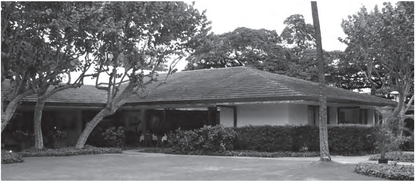
The Pacific Club (1959), designed by Vladimir Ossipoff, is an example of mid-century tropical modernism, which features key elements such as framing views, blurring the inside-outside connection, and use of natural ventilation and materials.
